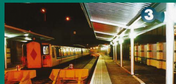
Opening of New Great Victoria Street Station. Autumn 1995
